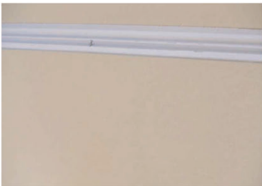
3) The wall is textured and finished, leaving a perfectly straight channel, ready to receive the fixture's reflector assembly.
